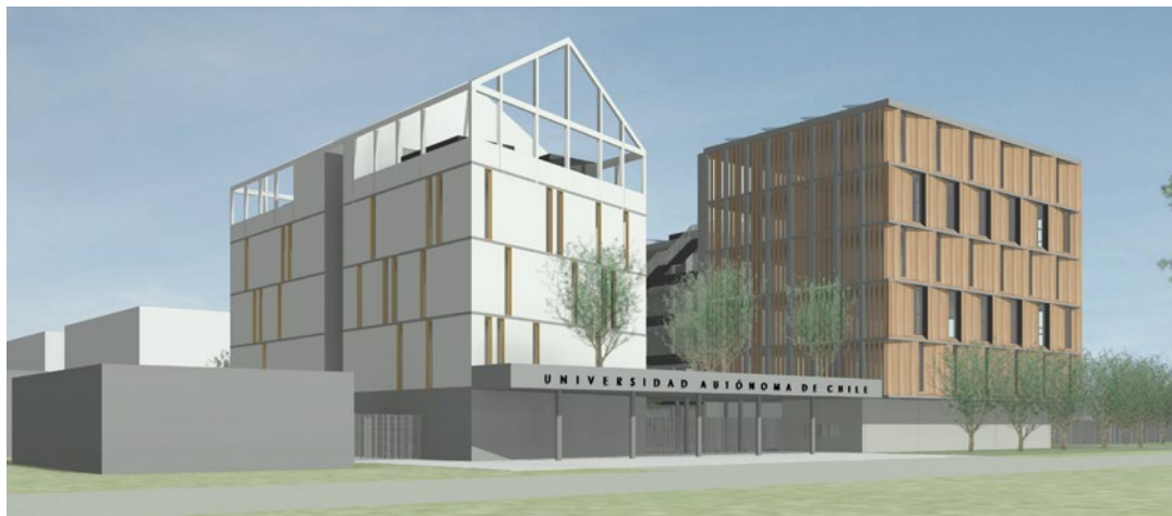
Campus Alameda Sur, vista nororiente
